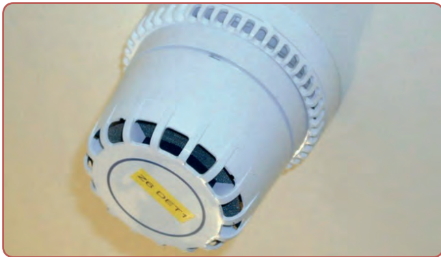
Figure 2-6-47: Smoke detector. Source: RMS.
