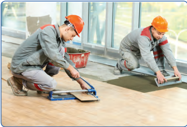
Figure 1-3-2: Contractors working at occupied premises. Source: Shutterstock.
