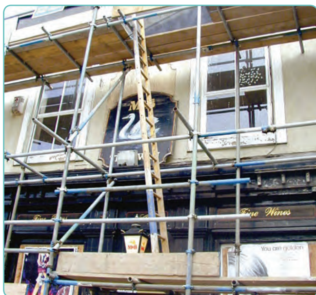
Figure 2-1-43: Independent tied scaffold. Source: RMS.
