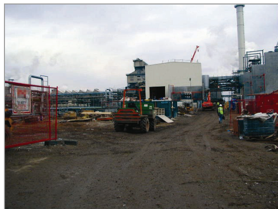
Figure 2-12: Site controls - access and roadways. Source: RMS.
