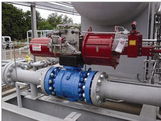
Figure 3-8: Emergency shut down valve.
