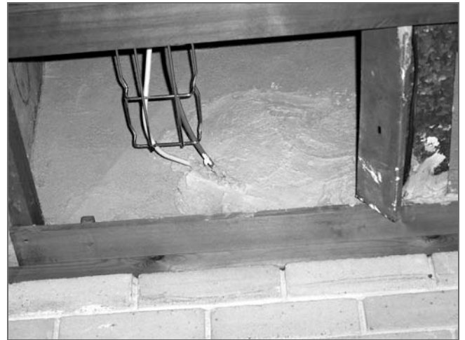
Figure 4-2: Fire stopping carried out correctly.
